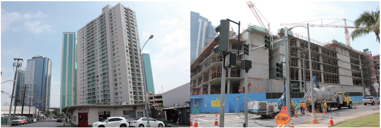
[Figure 9: Renovations of the Ward area]
