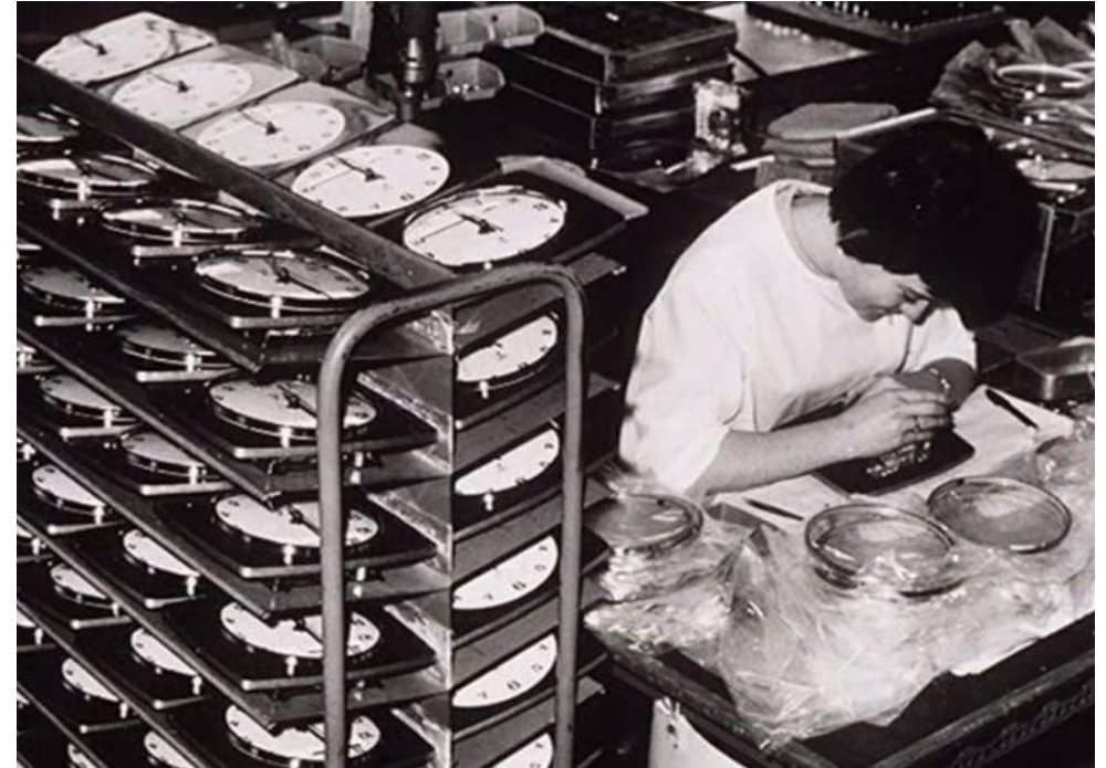
Assembly of radium luminescent paint alarm clocks
