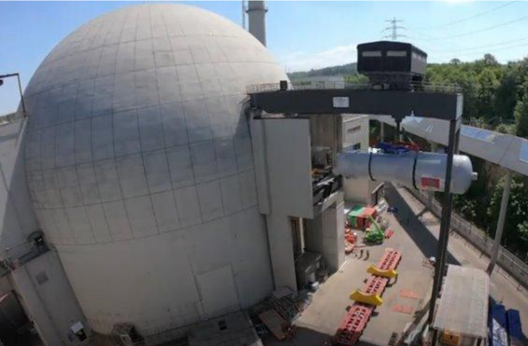
Neckarwestheim I NPP: Removal of steam generator in one piece Image source: EnBW AG
