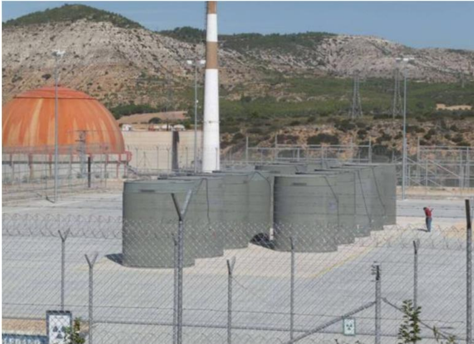
Dry spent fuel storage of the Jose Cabrera NPP, Spain
