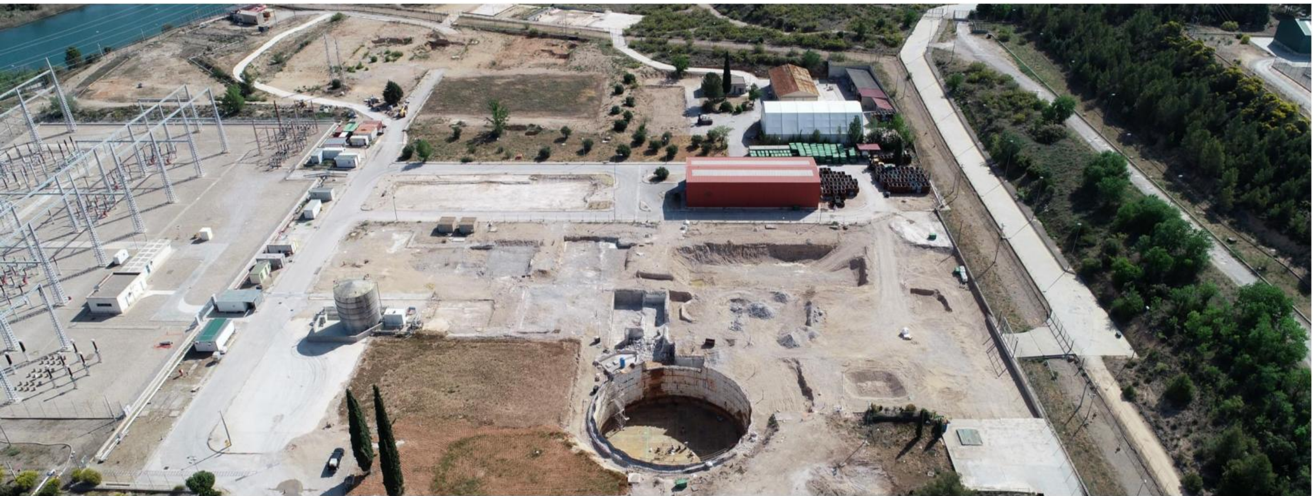
Jose Cabrera NPP site, Spain – as of May 2023
