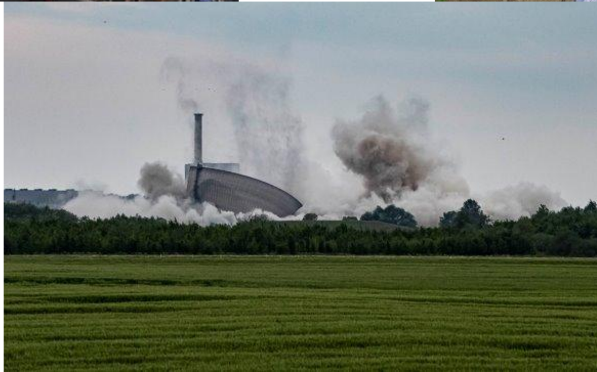
Philippsburg NPP: Blasting of cooling towers Image sources: EWN GmbH
