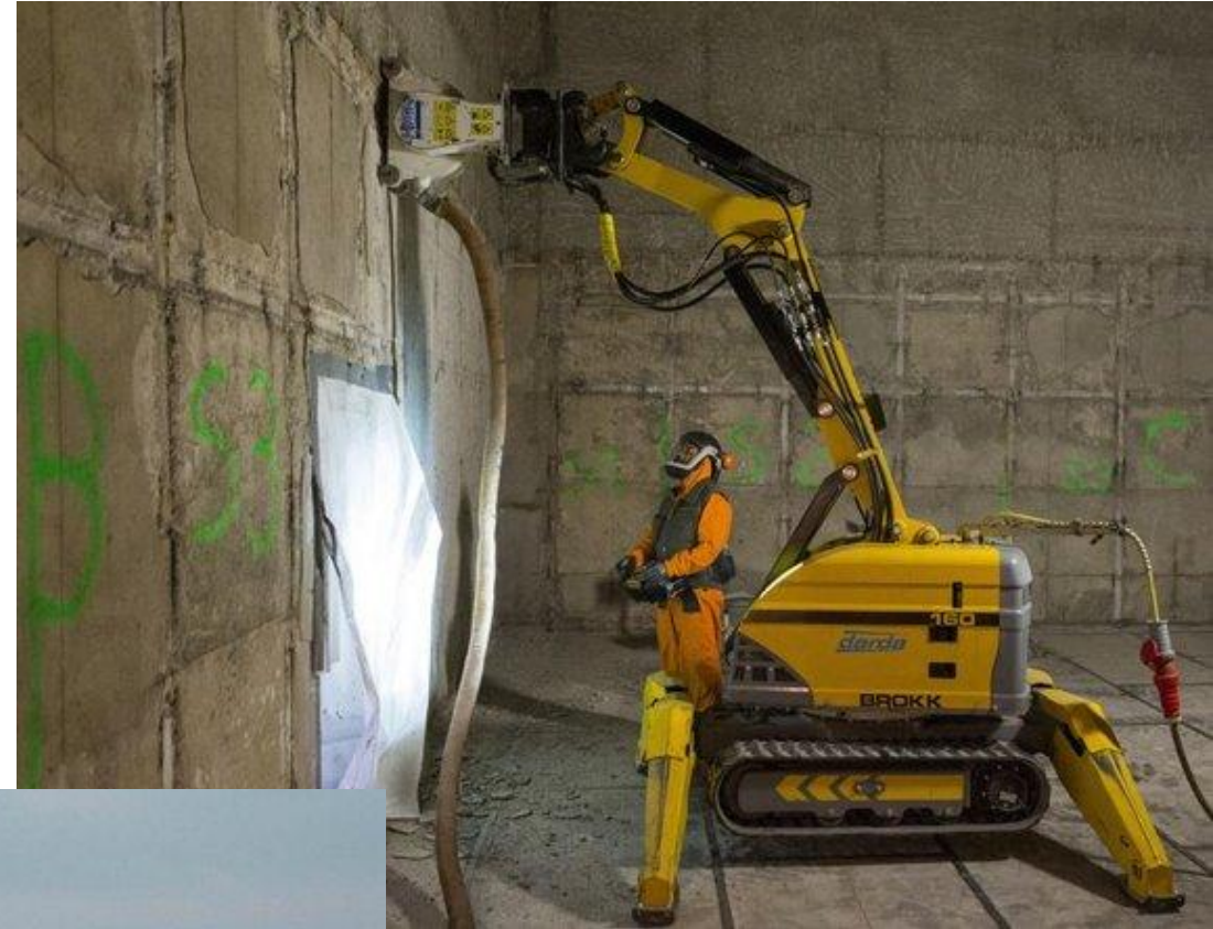
Greifswald NPP: shaving of concrete surface Image sources: EWN GmbH
