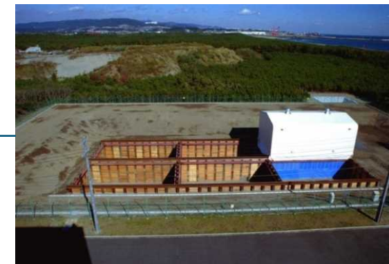
JAEA, Trench disposal (Tokai, Ibaraki)
