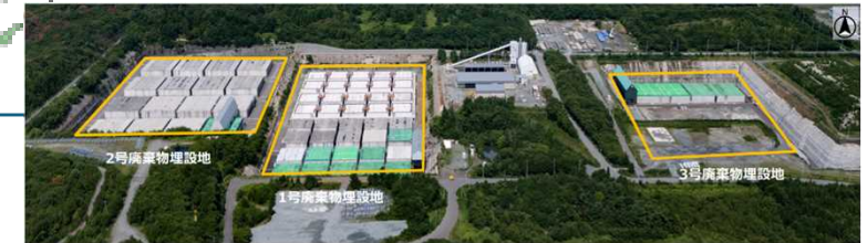
JNFL, Pit disposal (Rokkasho, Aomori)
