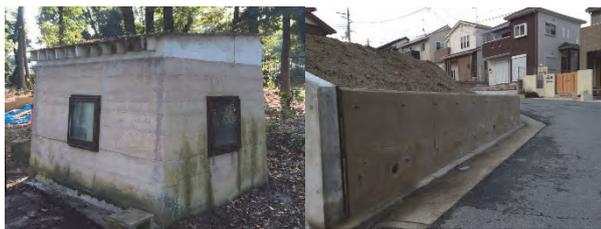
Fig.1 House and retaining wall using PVA fiber.
