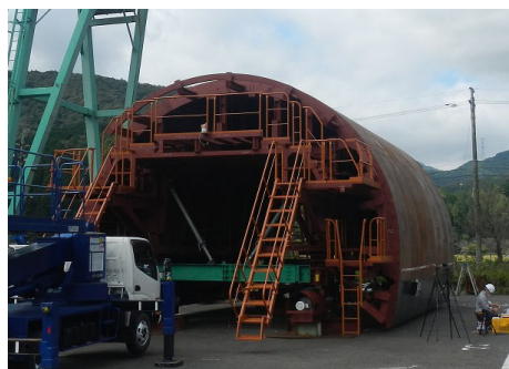
図 3. Centre for tunnel construction
